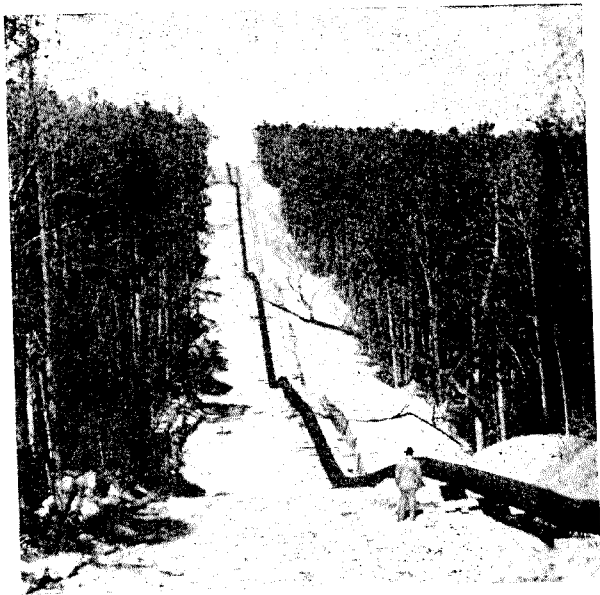
Somewhere along the route of the world's biggest oil line. This shows pipe on skids ready to be lowered into position.
