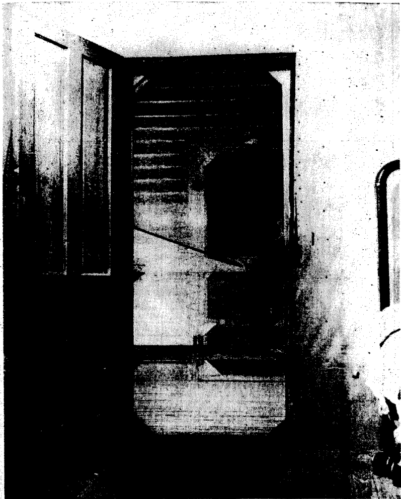
Fig. 7. House mosquito-proofing is an important aid in preventing malaria transmission. The above view shows a well-built screened door and walls covered with kraft paper.
