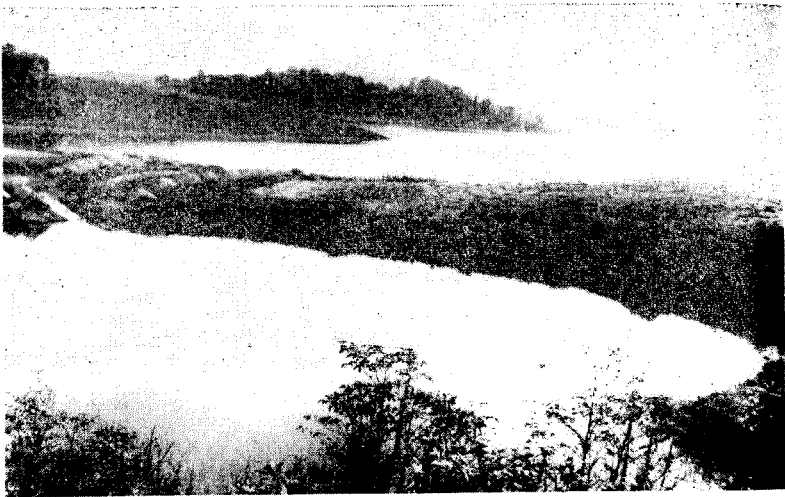
Fig. 2. Marginal drainage provides boat access to lateral depressions and makes it possible to regulate the water levels with those of the main reservoir. The above view shows a small limesink connected to the main body of a storage reservoir by means of a dragline ditch.
