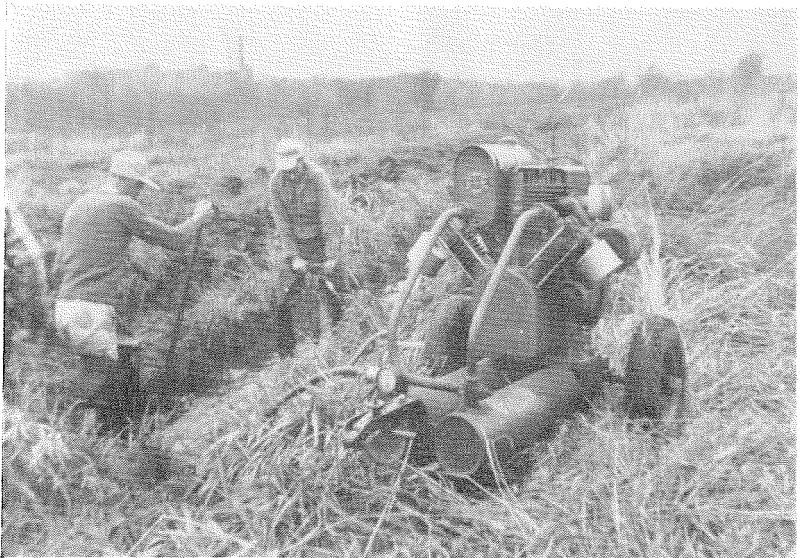
FIGURE 1. Light weight compressor used to facilitate ditch digging.
