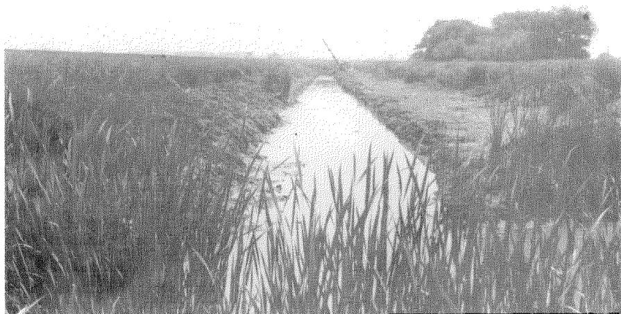
FIG. 1.—Marsh canal under construction
