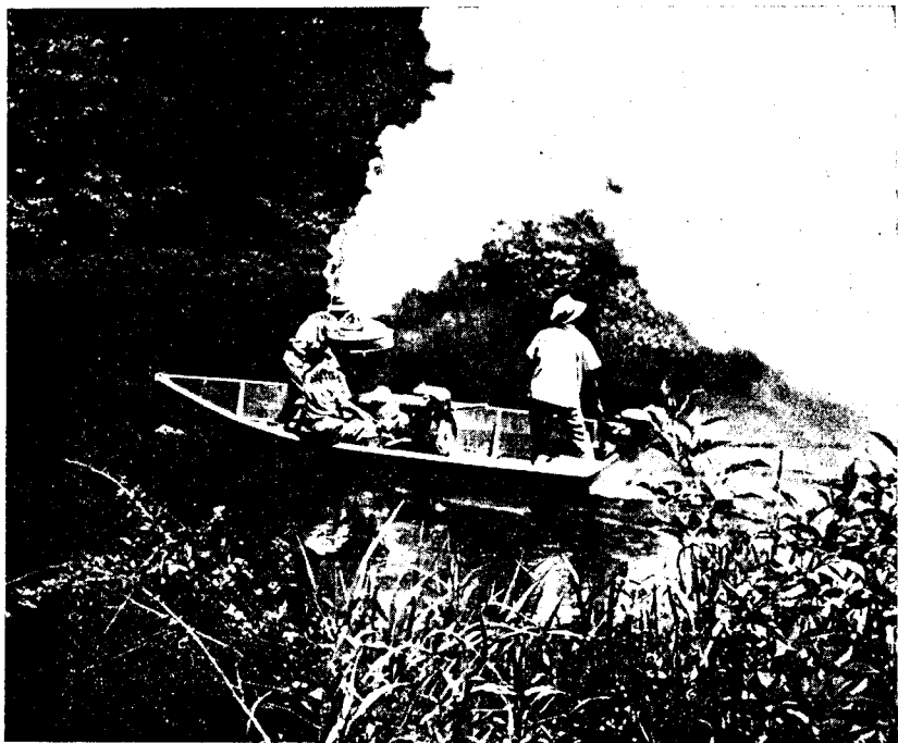
ENGINE-DRIVEN CENTRIFUGAL PUMP
