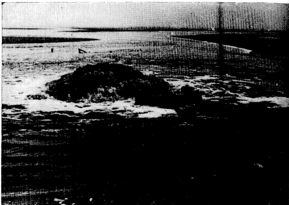
*Subterranean, "inverted siphon" outlet, Fishing Creek Marsh, Cape May County, New Jersey. Discharging at extreme low tide. Exposed to direct wave action from Delaware Bay, but not damaged by the recent hurricane. Type two outlet is used here because bay is very shallow and at low tide, sand bars (dark areas in background of photo) are exposed for a distance of more than 1,000 feet and length of pipe for a type one outlet would be excessive.*
