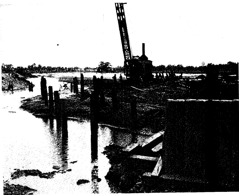
Fig. 2. Navy Drainage Project for Elimination of Mosquito Hazard, Boush Creek, Norfolk, Virginia. Intake end of 24 foot canal. Two lines of wooden piling will be cut off to carry reinforcements for concrete floor while cross piling near machine will brace wing-wall.
