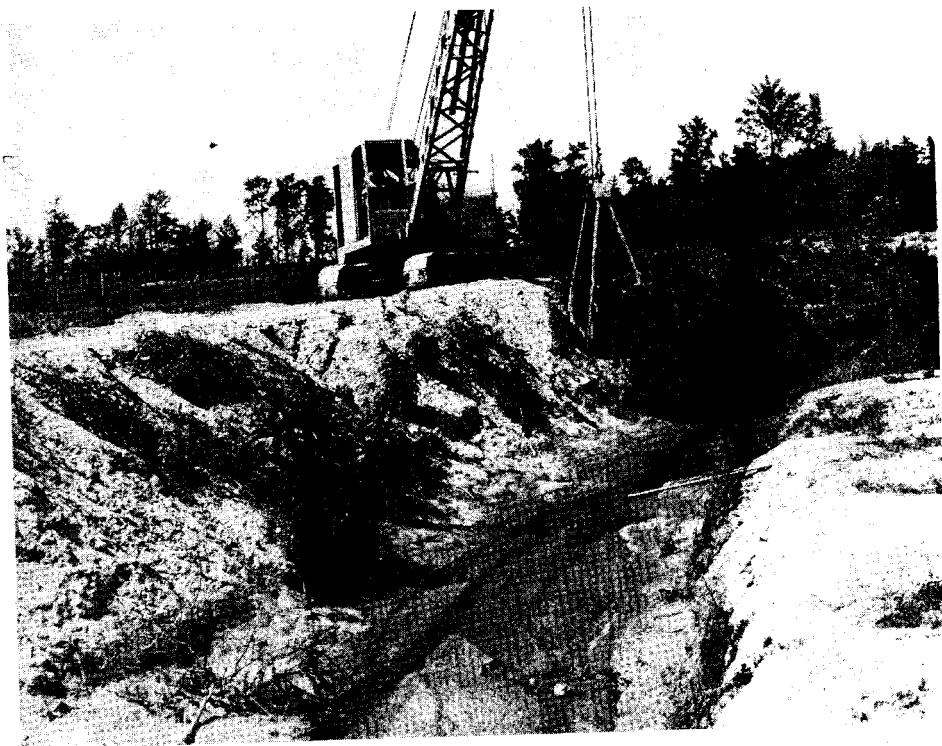
Fig. 4. Navy Drainage Project for Elimination of Mosquito Hazard, Boush Creek, Norfolk, Virginia. Several ditches, like the one being reconditioned here with a bucket-crane, will carry surface run-off to piped openings in the side walls of the 24 foot canal.
