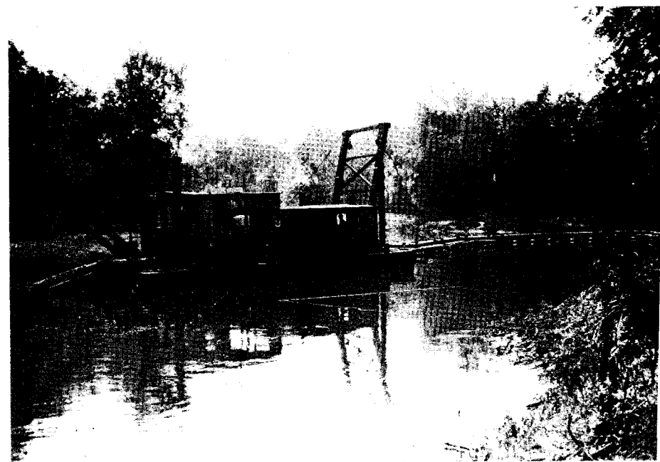
Fig. 1. A specially designed, sectional dredge-boat used in inter-county, mosquito control improvement of the upper Passaic River.
