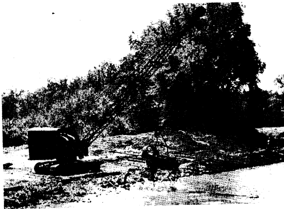
Fig. 5. A \frac{3}{4} yard drag-line bucket operating from a caterpillar crane equipped with a 40 foot boom
