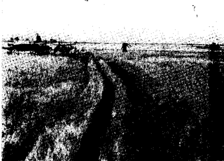
Fig. 3. Photograph illustrates work completed by a special 10" marsh plow which was developed by the State Highway Department. It is used largely for connecting breeding pools to lateral ditches.
