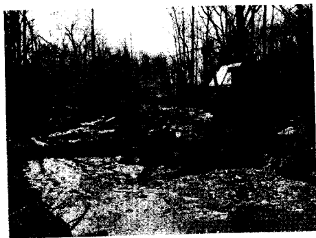
Fig. 1. Hackensack, New Jersey, February, 1942. Power shovel with \frac{1}{2} -yard drag-shovel attachment. Clearing the channel of a brook through a woodland swamp.
