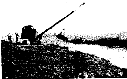
Fig. 4. Moonachii Creek, March, 1943. Power shovel with \frac{3}{8} yard dragline bucket, cleaning large drainage creek on salt marsh.
