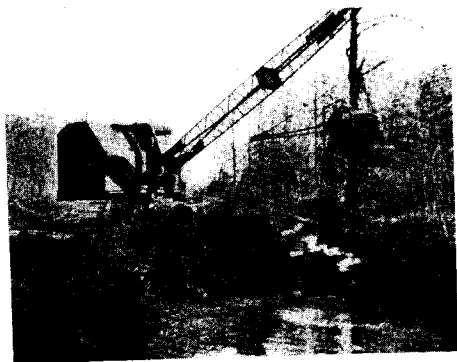
Fig. 3. East Riser, New Jersey, January, 1943. Power shovel with \frac{1}{2} yard dragline bucket widening the channel of a brook from 5 feet to 12 feet for flood control.
