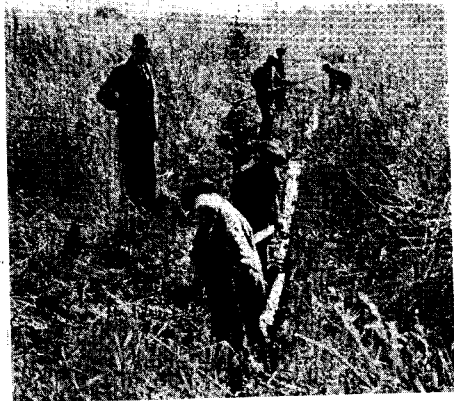
Fig. 2. Reconditioning a mosquito control ditch on a Monmouth County salt marsh.
