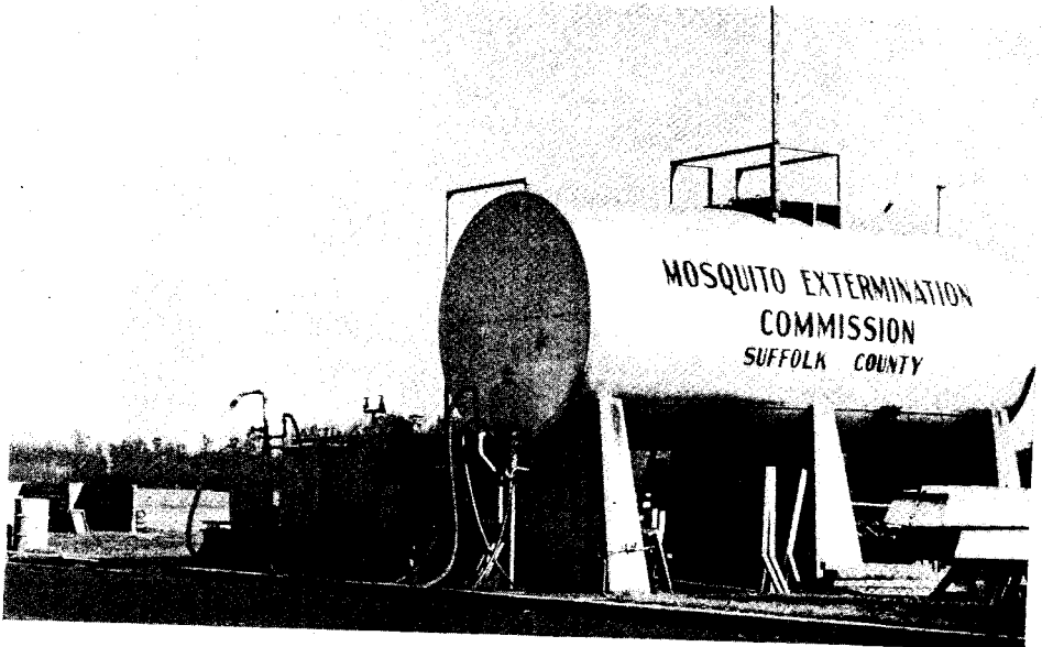
Fig. 3. Storage tanks for oils and larvicide materials.
