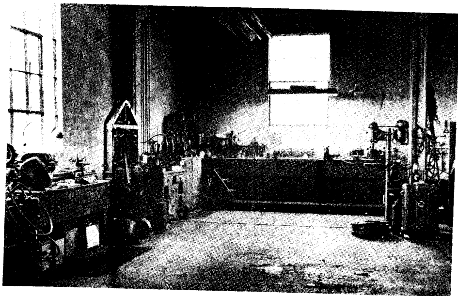
Fig. 6. Machine shop for servicing mechanized equipment.
