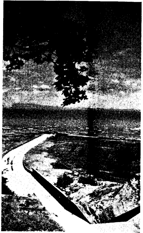
FIG. 4. Terminal spillway and chute.
