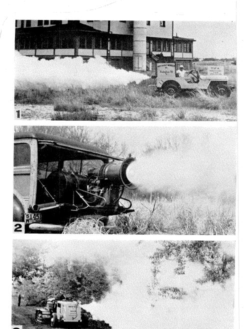
ial deposit could be demonstrated as far s 200 feet from the machine. The coarser Tession mist is much less influenced by tmospheric conditions and provides the hearest approach to airplane treatment with ground equipment.
