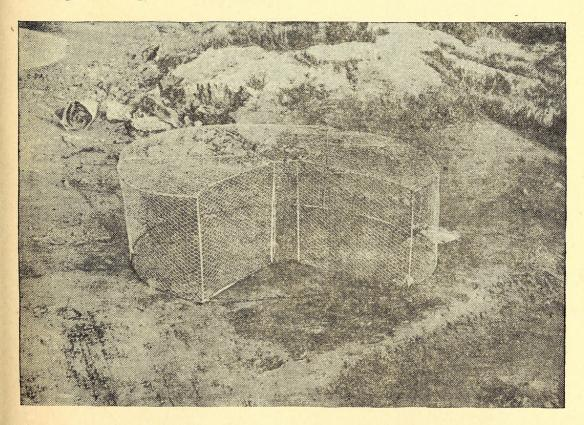
The size of the traps is about 1 m. 80 cm. in diameter by about 65 cm. in height. The framework is made of stout galvanized wire
