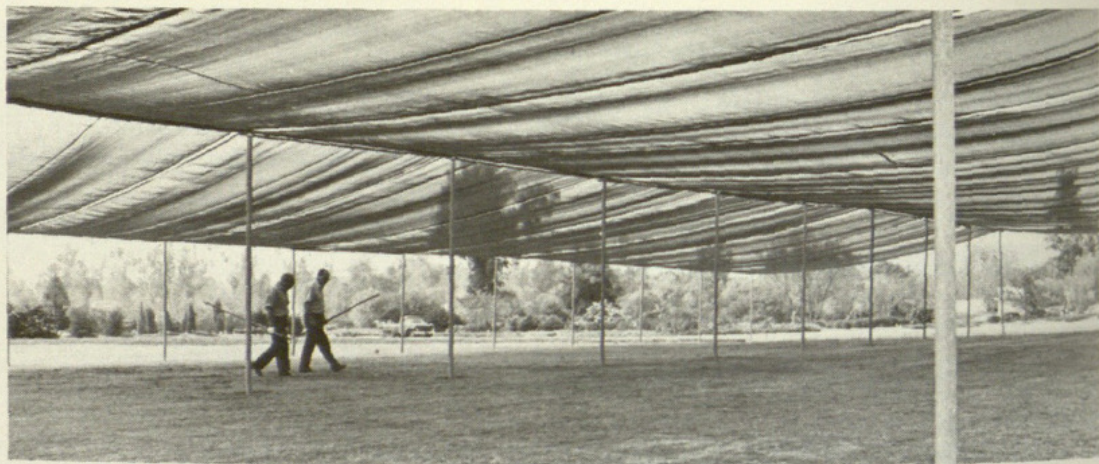
This 6,000-square-foot shade area at the Arboretum was built to provide cover for outdoor events. It is designed so that the saran-covering can be put up or taken down easily and quickly according to the weather and the requirements of the event.
