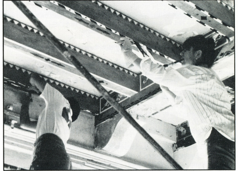
Artisans restencil Moorish designs on ceiling beams.
