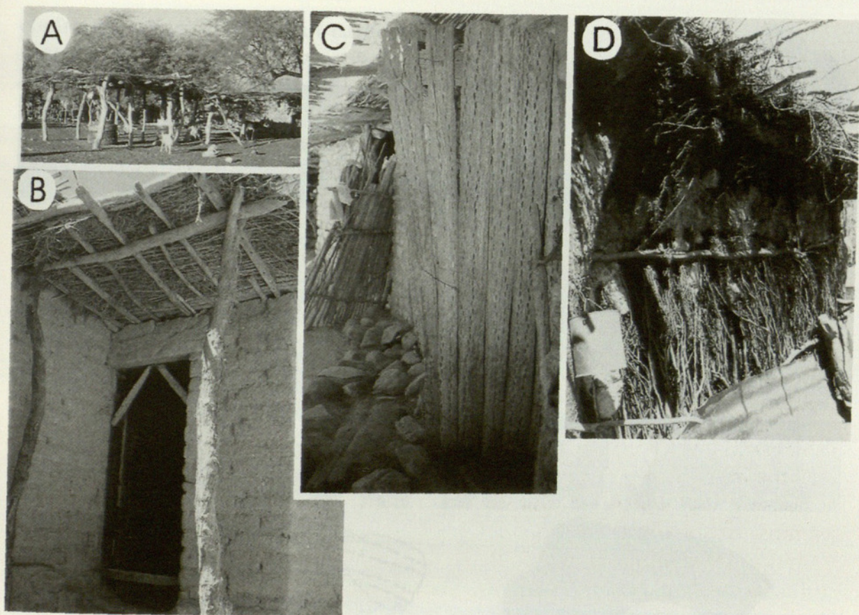
FIGURE 2.—A traditional house at the Hualfin Valley. Different types of construction could be observed at the same habitation area for an extended family: a) wooden structures for shading and drying Prosopis fruits; b) adobe bath room; c) stone room; d) twig kitchen.
