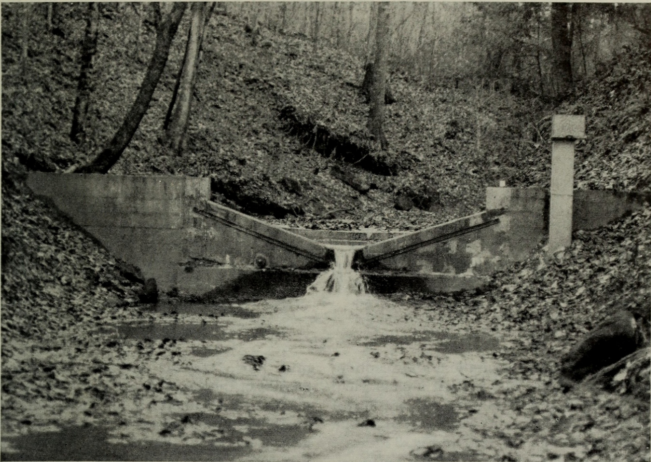
FIG. 2. V-notch weir used for measurement of streamflow.
